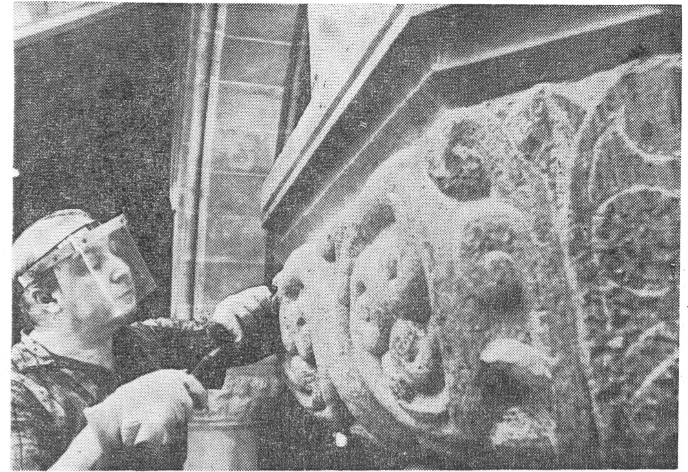
ART IS HARD WORK —Marozzi uses a pneumatic chipping gun to carve flowers in stone.—Photos by Warren Roll.
